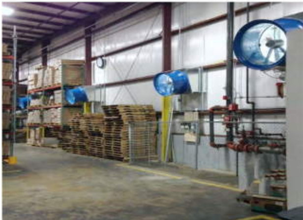
High Velocity fresh air intake systems
