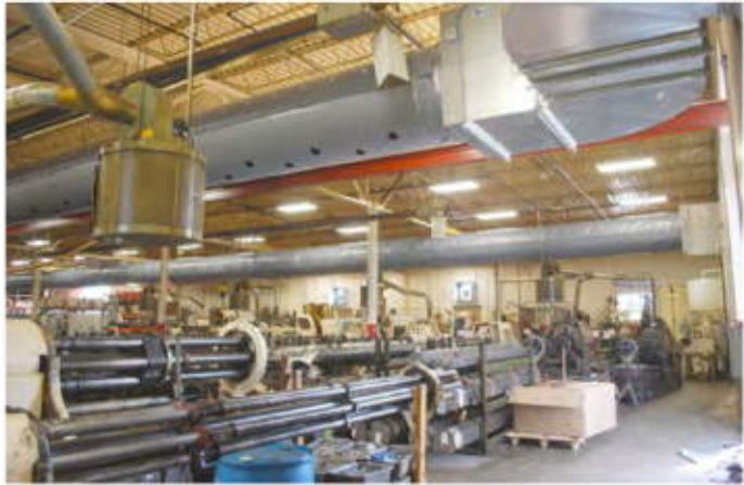
Quietaire fabric ducted fresh air make up
