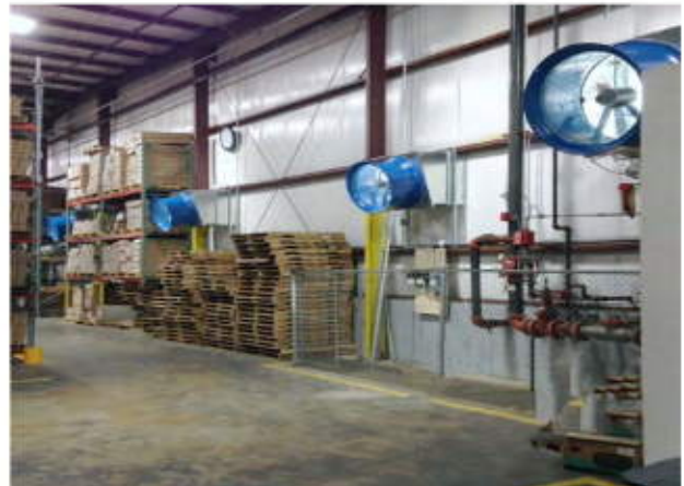
High Velocity fresh air intake systems
