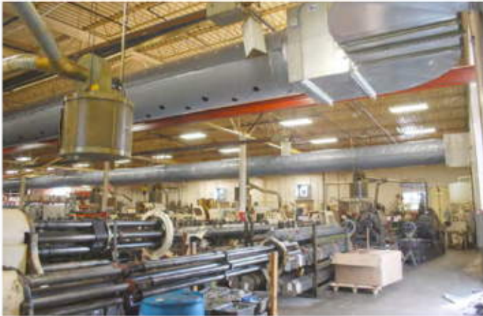
Quietaire fabric ducted fresh air make up
